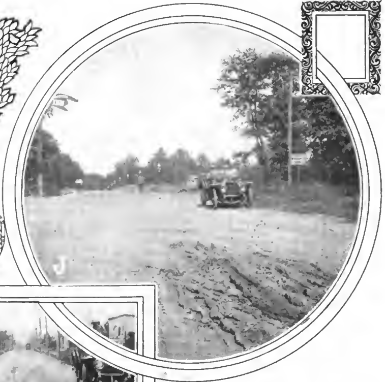
H—Another example of a road surface running parallel to that shown in Fig. G, but with a surface so soft that even a person's footprint makes an impression on the surface. The road shown on the right of the picture is being prepared for a tar surface
